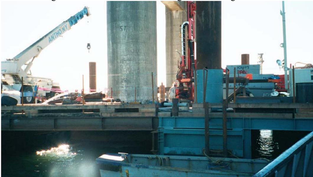
**Figure 3.** Pier 57 Production Pile work platform. The boat in foreground is docked in front of the metal frame with buoyancy tank that made up the majority of the work platform structure. The work platforms were pinned-off to 24 inch diameter driven pipe piles (shown in the background) at the highest tide to minimize the influence of tidal changes on platform motion. The pier's concrete columns are shown at the center of the picture.
